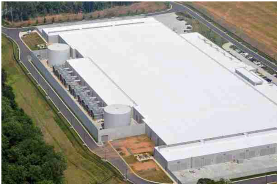
Apple's data center in Maiden opened in 2010. At 505,000 square feet, it's the biggest data center in the state, with capacity for 100 MW.
